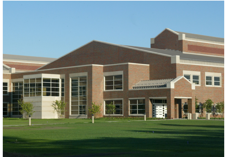
Central Michigan University's state-of-the-art Health Professions Building incorporates education, research, and clinical practice into one facility, and facilitates sharing among faculty, students, researchers, and practitioners.
